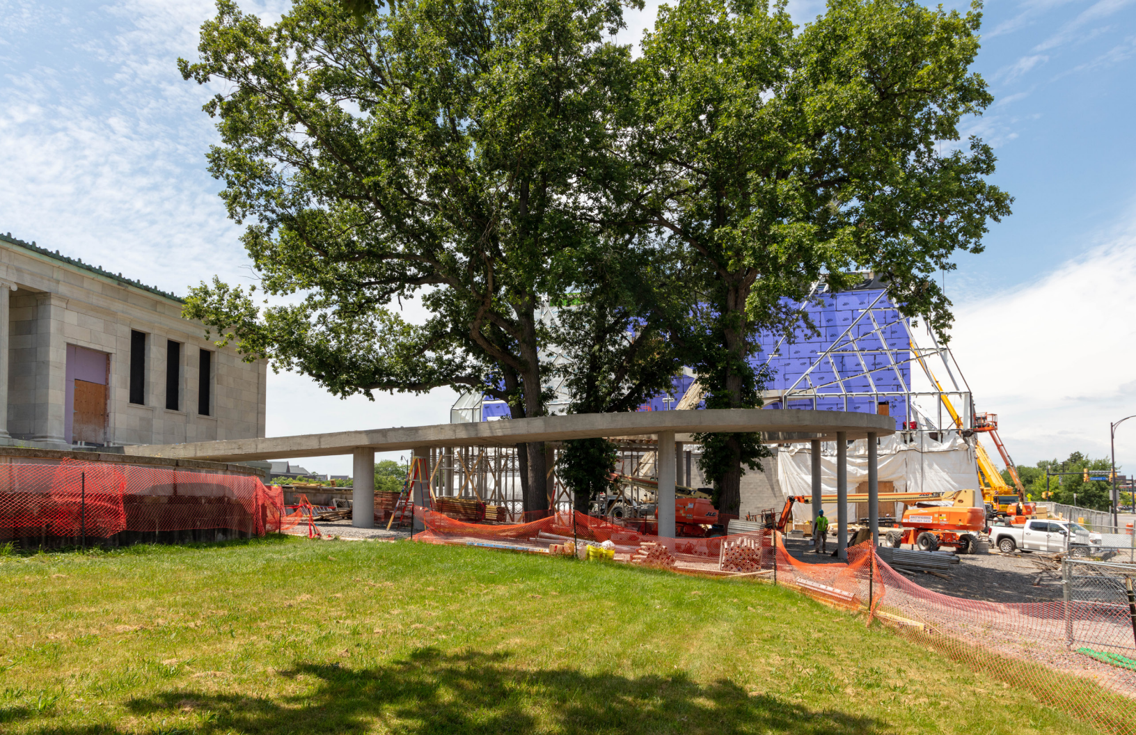
The foundation of the John J. Albright Bridge. Photo: Jeff Mace
